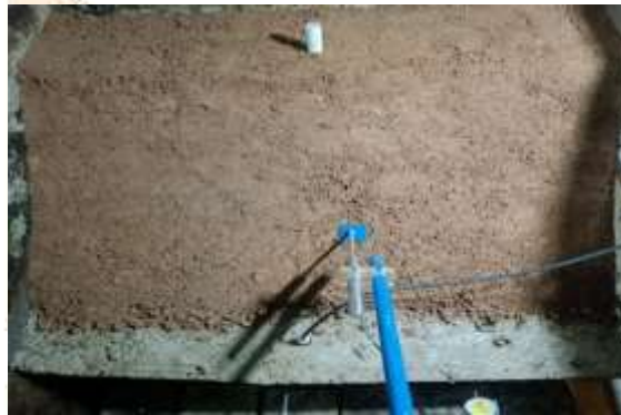
Fig.3 Stage-wise construction of embankment
