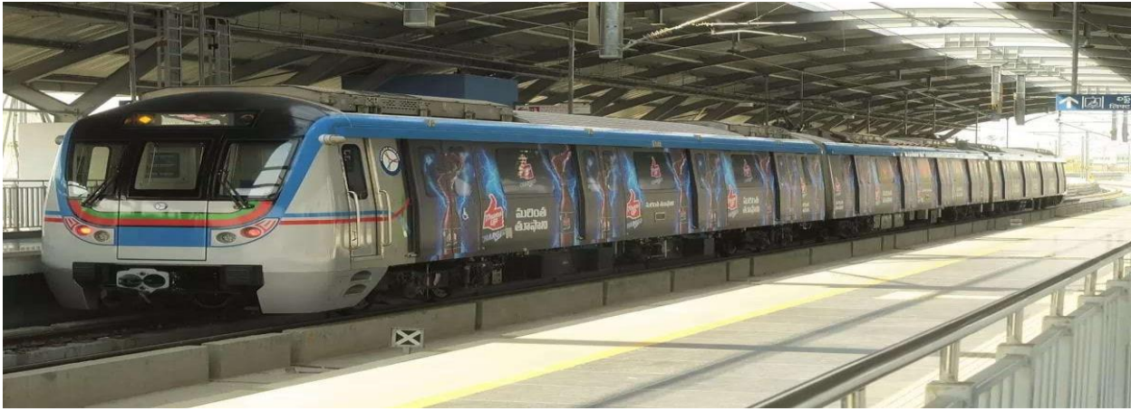
Figure 1.1 Nampally Metro Station
